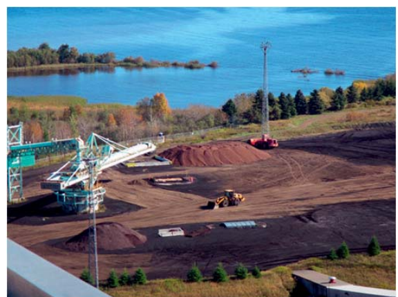
View of the fuel yard (Copyright of photo: Ontario Power Generation)
