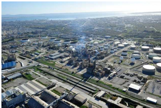
Figure 3: The Thessaloniki refinery of Hellenic Petroleum in Greece: case study site for HVO production
