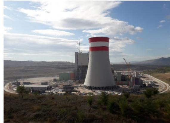
**Figure 5:** The Ptolemaida V 615 MWe lignite-fired power plant (under construction). Due to the 2028 Greek Coal phase-out, a bioenergy retrofit is one of the options considered for keeping the plant operational.
