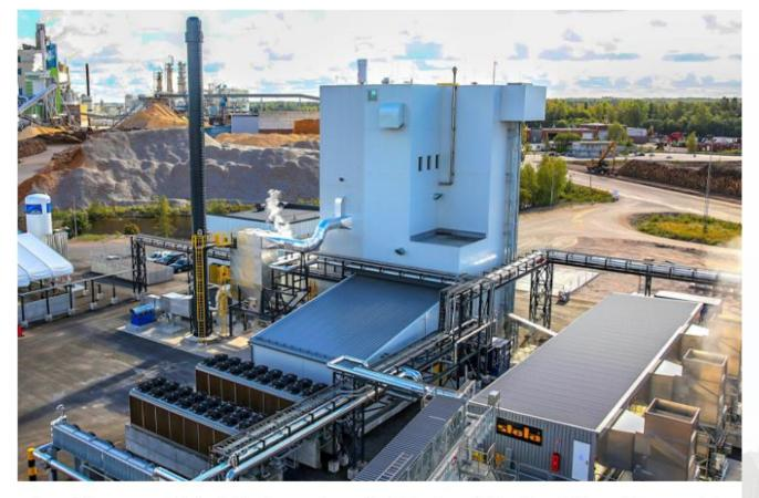
Preem AB has announced that production is now underway at its joint venture subsidiary Pyrocell AB's novel biomass pyrolysis plant in Gävle. Using pyrolysis technology, the pioneering plant converts sawdust into bio-oil which is then used as a bio-crude for processing into renewable fuels at Preem's Lysekil refinery (photo courtesy Preem).
