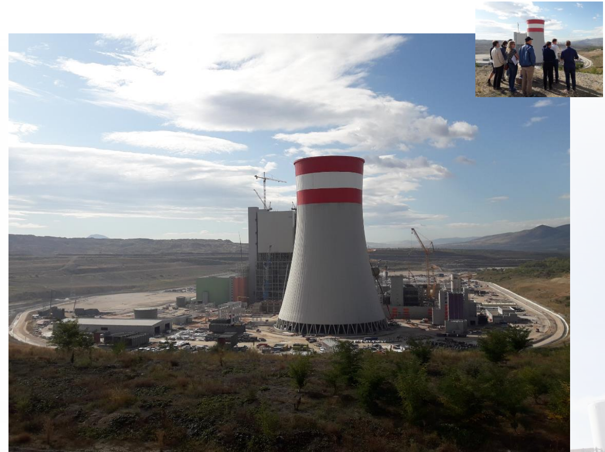
Ptolemaida V 600 MWe power station (under construction), Due to the 2028 Greek Coal phase-out, a bioenergy retrofit is considered.
