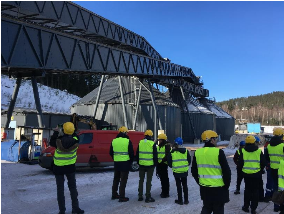
Figure 4. Coal is used only if the peat and wood conveyors do not work.
