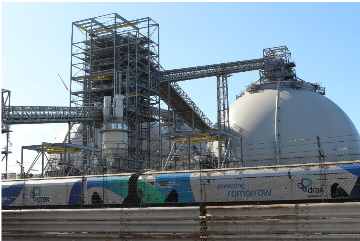
Figure 6. Close-up of the biomass domes and train wagons used at Drax for wood pellet storage and transport respectively.
